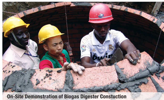
On-Site Demonstration of Biogas Digester Construction
